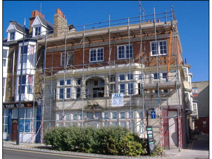
Metal scaffolding encasing the same building – September 2007
