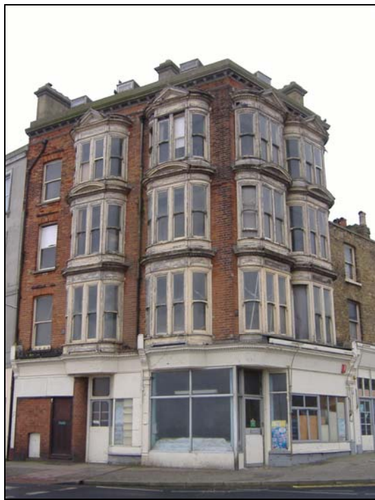
Now looking sad and neglected
